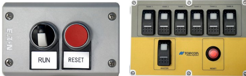
Run/Stop switchbox (A1771)
